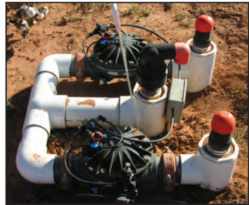
Figure 3. Example of a field installation of pressure regulating valves and air vents
